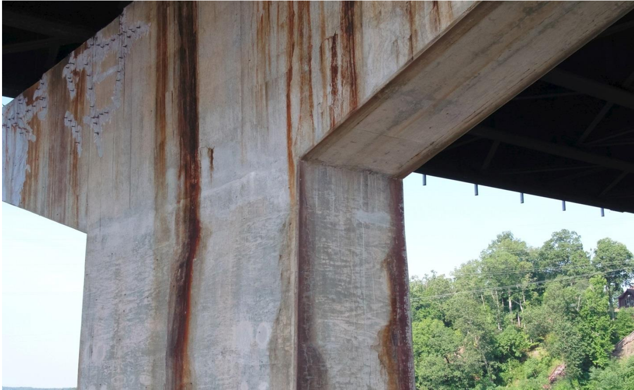
Figure 3. Single Photograph of Bridge Pier Captured from UAS
