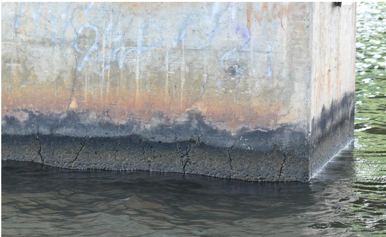
Figure 4. Single Photograph of Pier Base at Waterline Captured with Handheld DSLR Camera
